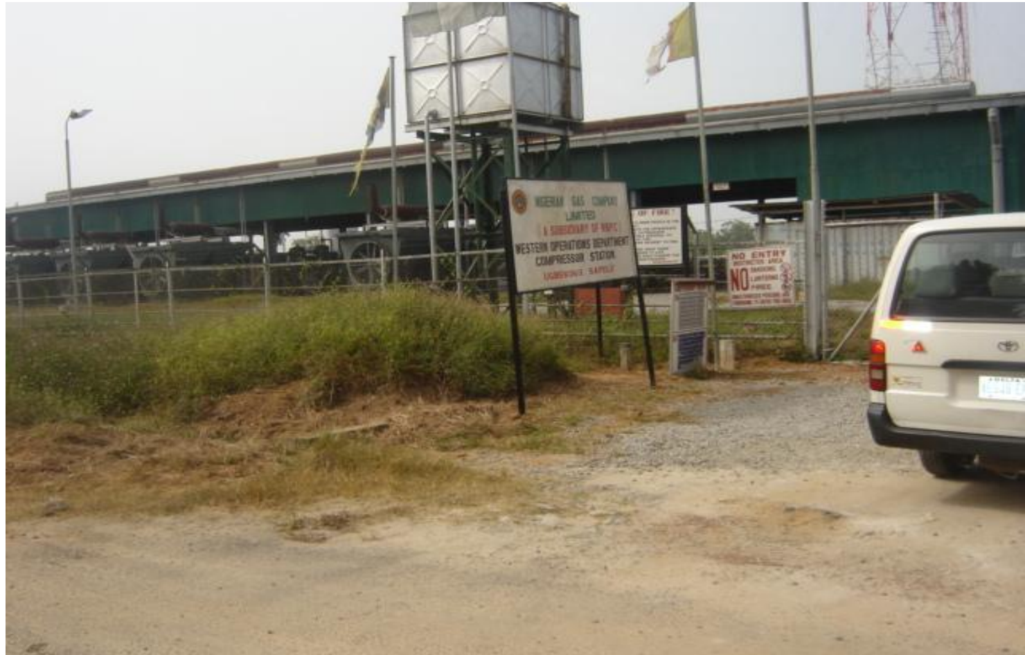
COMPRESSOR HOUSE – SIX INGASOL RAND AND CAT. ENGINE DRIVEN
